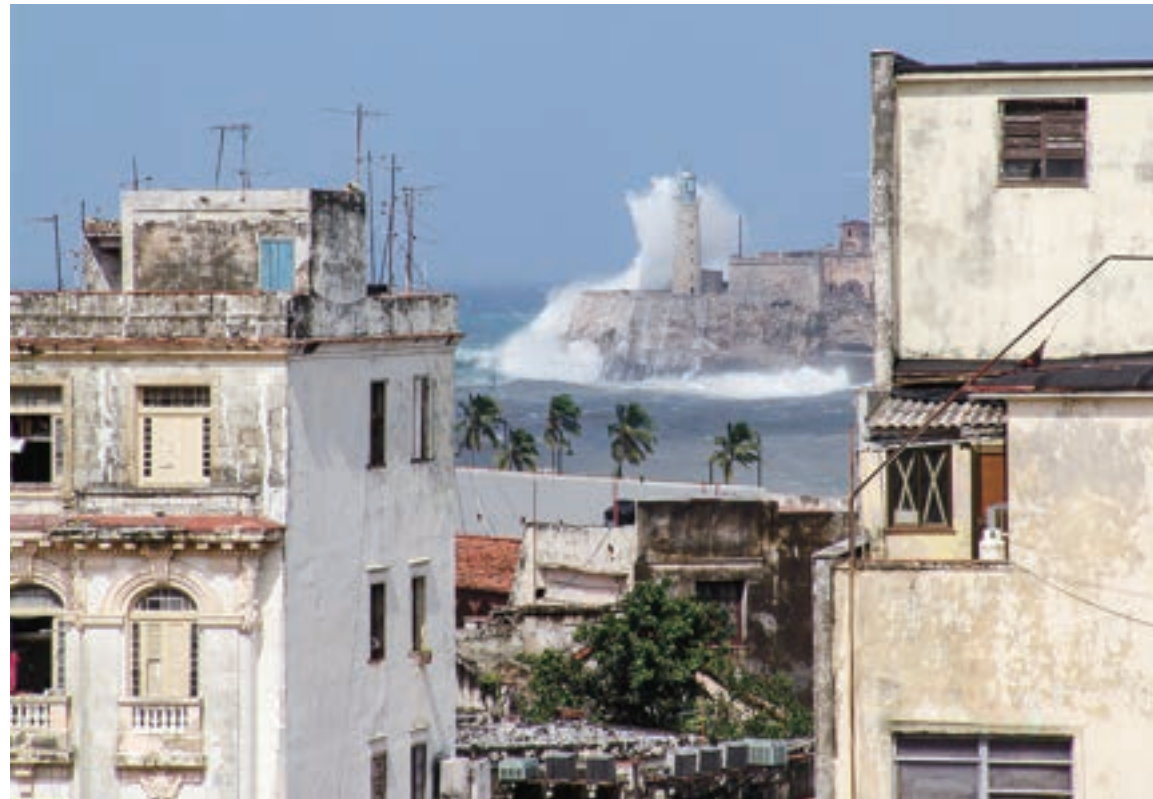
Hurricane damage is visible with Castillo de los Tres Reyes del Morro in the background.
