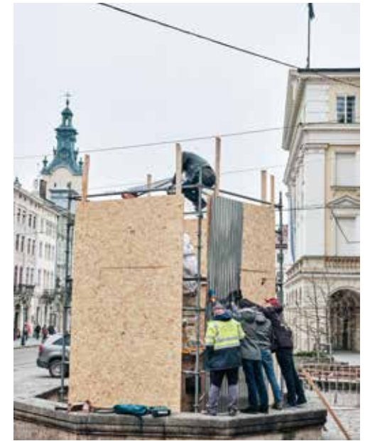
Lviv. Protective structure. Fountains in Rynok Square March 2022. Photographed by Vasyl Rohan
